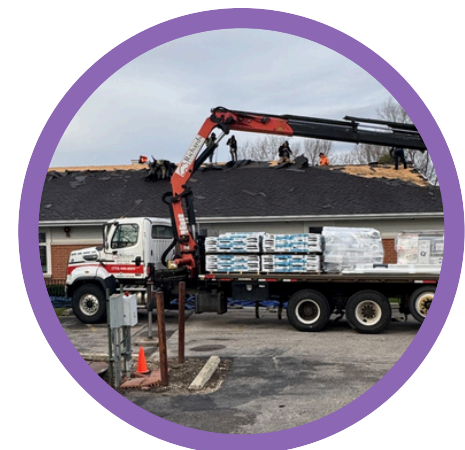
Peerless Roofing did a phenomenal job replacing our shelter roof!
